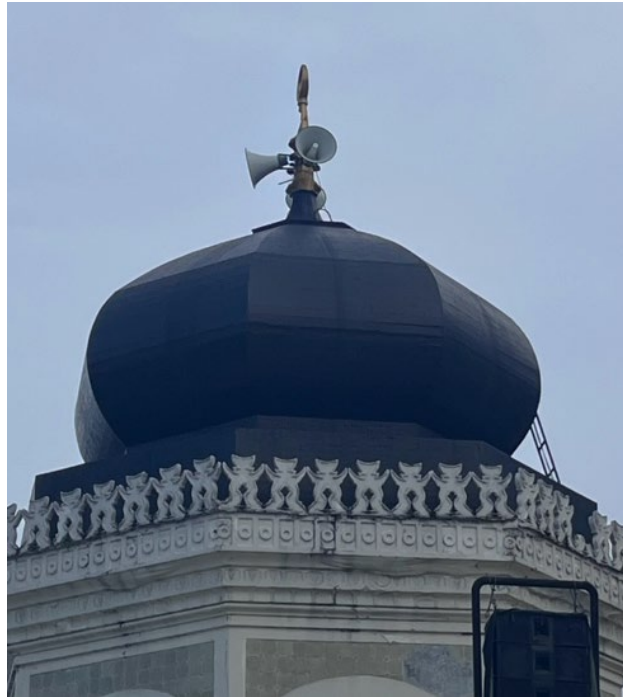
Figure 1 Use of horn speakers installed atop a mosque dome in Medan (North Sumatra) as part of a sound system for the call to prayer and religious announcements.
